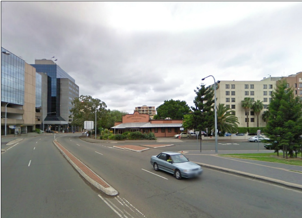
Photograph 1 shows the existing building on the site as viewed from Parkes Street looking east.
